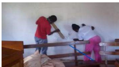
Inside the church preparation work
